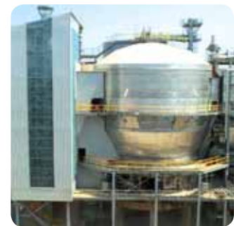
Roasting over 300,000 tpa of Zinc concentrates in a 123 m 2 fluidized bed.
