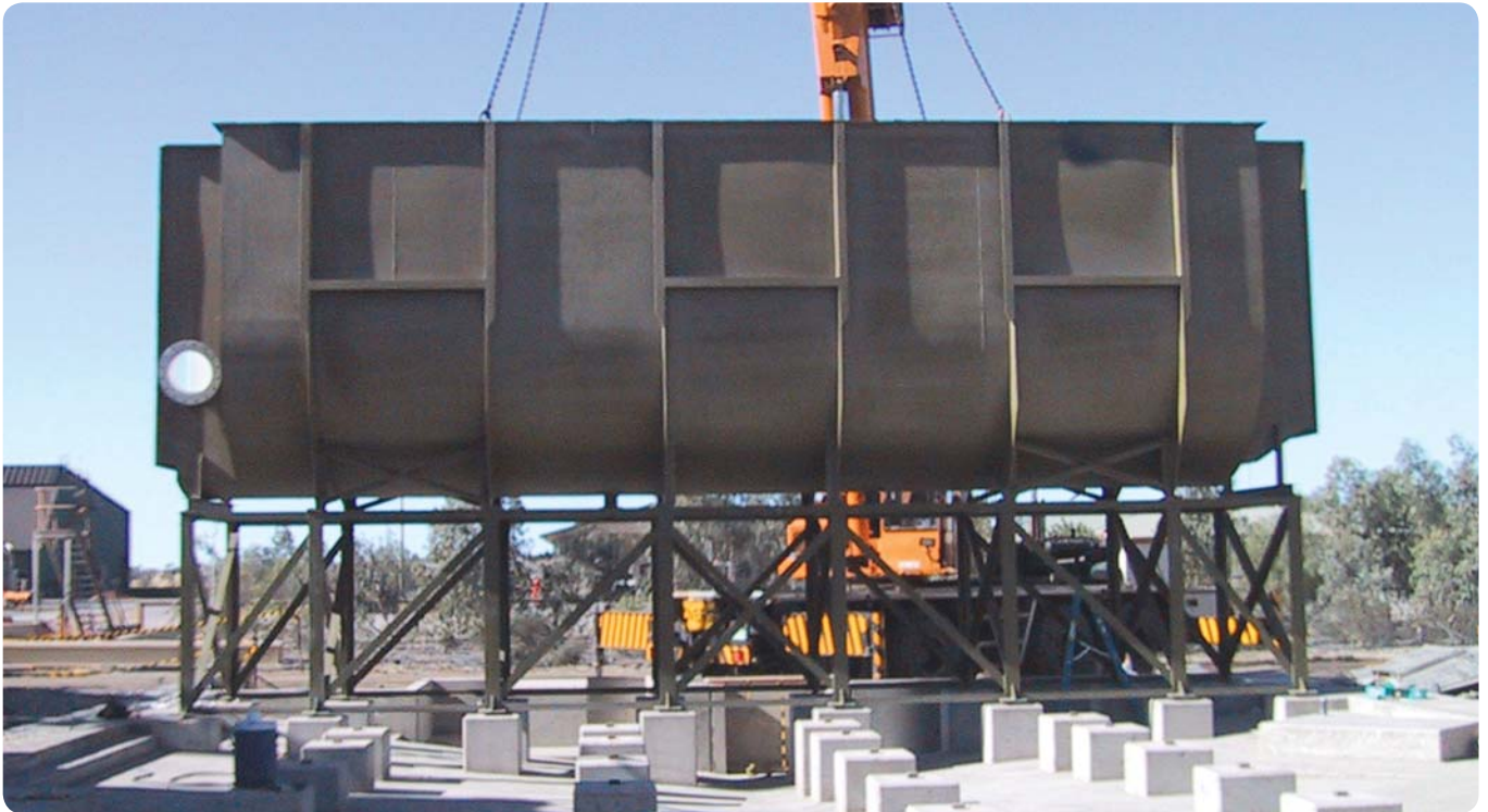
Installation of tank and support structure for zinc cleaner 3.
