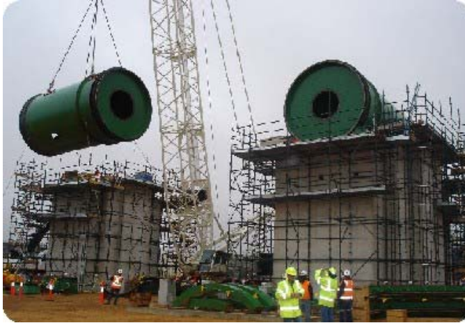
Installation of scrubbers at Ravensthorpe
