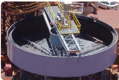
High rate thickener – low sidewall depth
