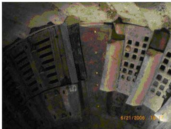
TPL™ system on the left and old radial pulp lifters system on the right.
