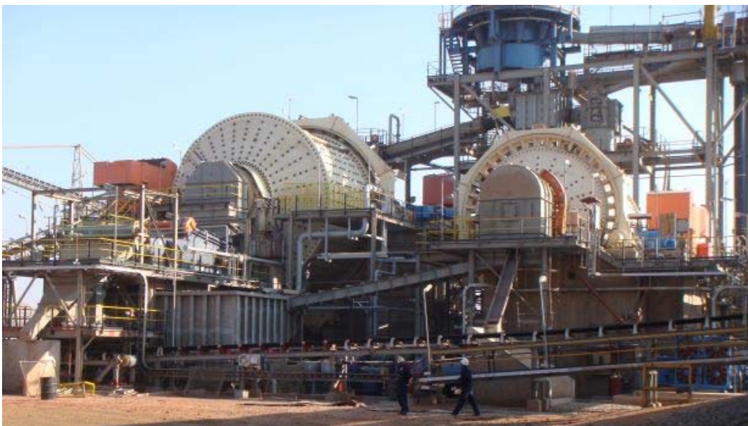
Final commissioning of Kansanshi's 12MW SAG and 5.8MW Ball mills
