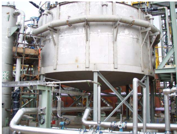
An Outotec 7.1m stainless steel HCT thickener
