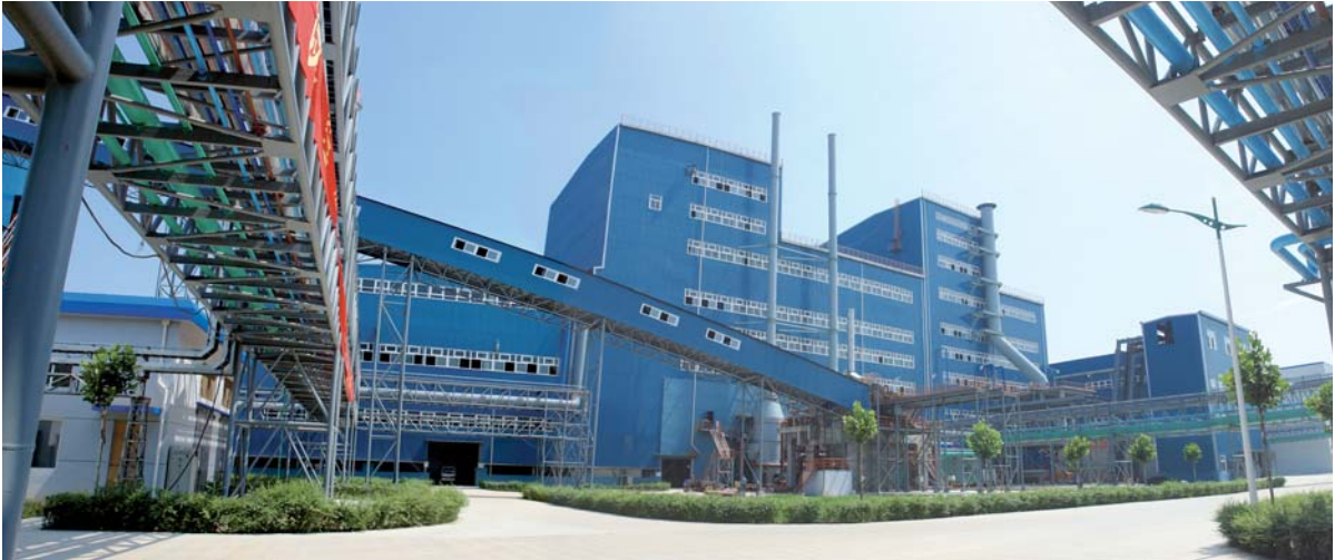
Yanggu Xiangguang copper flash smelting and flash converting plant, China.
