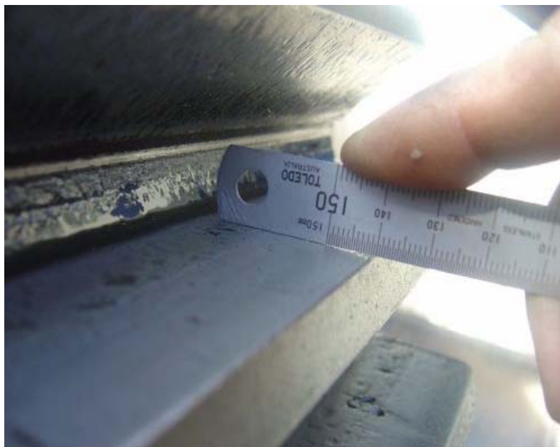
Mill ring gear inspection, worn gear tooth profile
