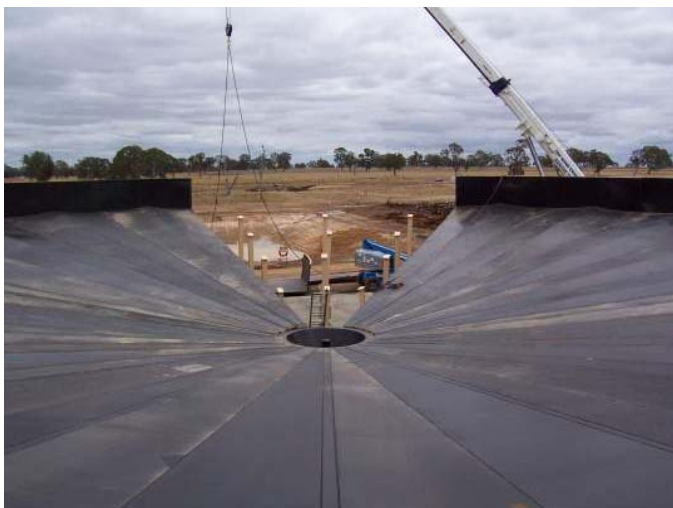
Floor gores installation
