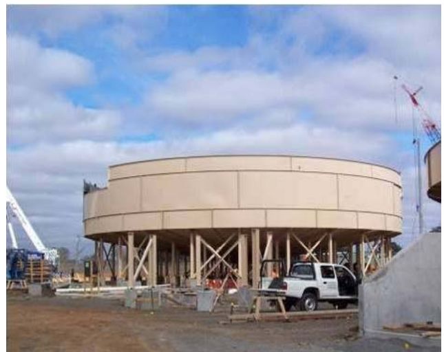
Tank walls almost completed & joints sealed
