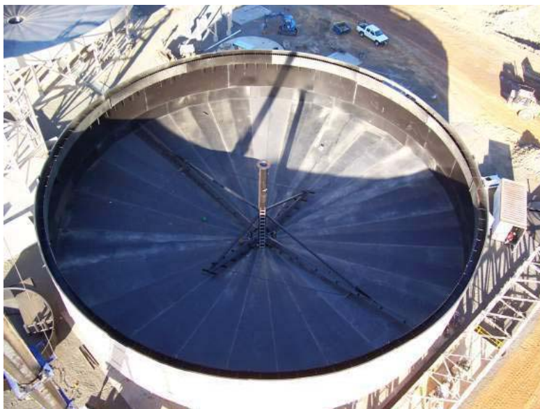
Rake mechanism assembled in bottom of tank
