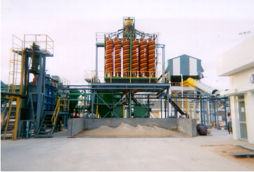
Figure 3 St. Gobain Glass Sand Plant
