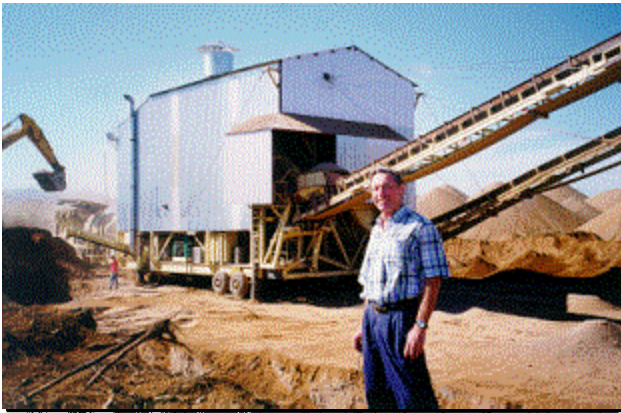
Photograph 3. Enclosed Dry Process Plant and Tailing Conveyors
