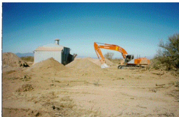
Photograph 1. Mobile Dry Process Plant with Tracked Back-Hoe Excavator
