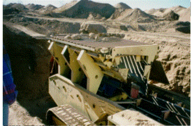
Photograph 5. Grizzly/Hopper with Apron Feeder
