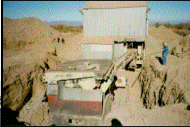
Photograph 2. Grizzly and Plant Feed Conveyor
