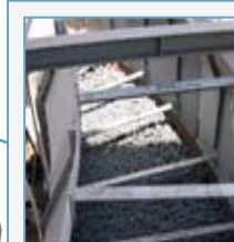
Tata Steel Iron ore sintering technology
