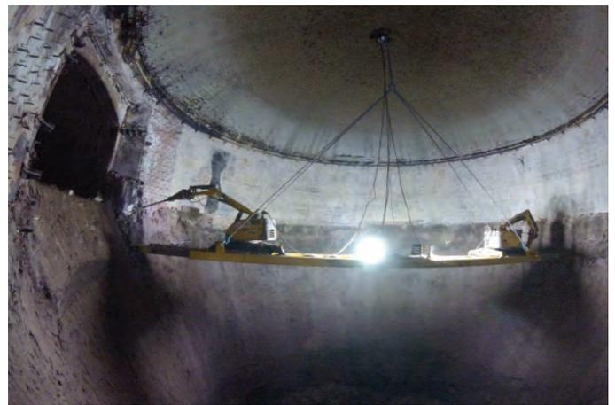
Outotec Roasting Refractory Demolition Platform on upper vertical wall
