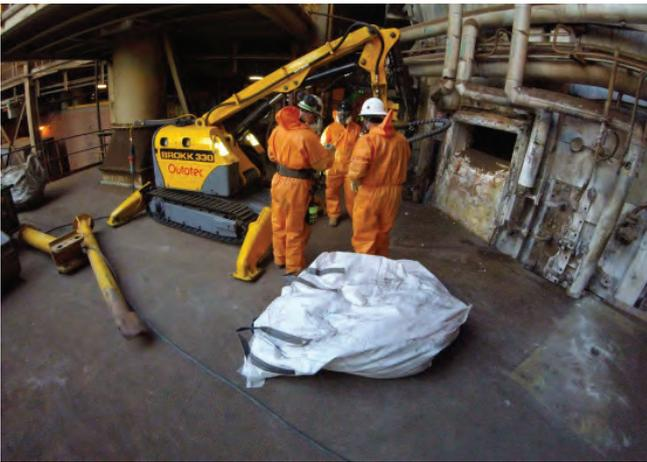
Outotec remote demolition robot machine and experienced operators
